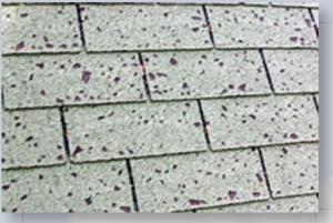
High winds can tear and remove shingles from your roof, leaving the roof deck exposed to the elements. A sudden drop in temperature combined with moisture in the air can cause storms that pummel your shingles with hail. Dents and pockmarks result, stripping shingles of the protective granules that guard against rain and sun damage.
